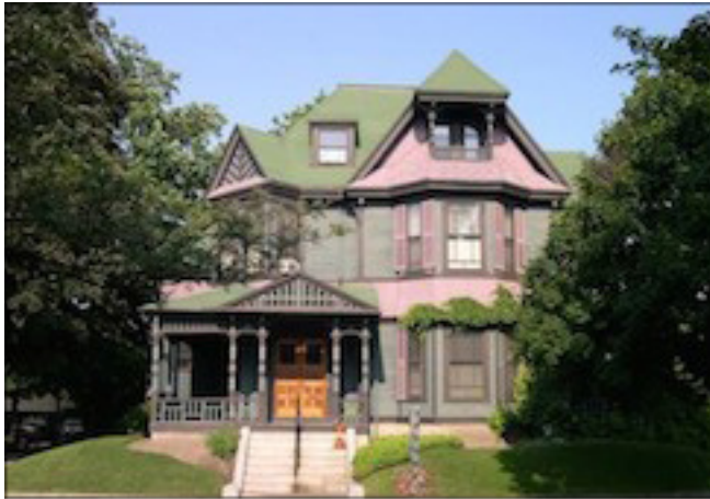
44. Andrew Gerrish, Jr. House
